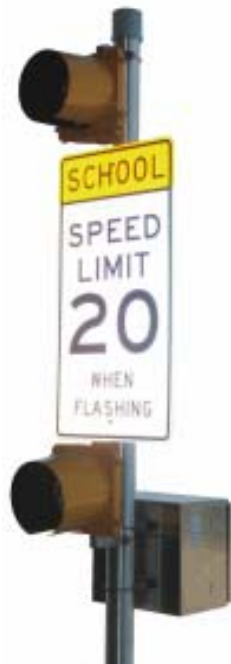
Flasher Cabinet Assembly (with AP22 Time Switch shown)
